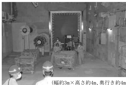
Fig.9 Transfer route newly developed by boring an opening through concrete wall
