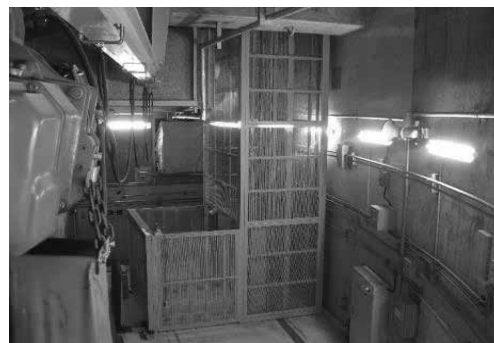
Fig.10 Installation of Vertical conveyor
